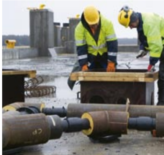
Pre-insulated Wehotek piping provides water service for ships at Vuosaari Harbour in Helsinki.
