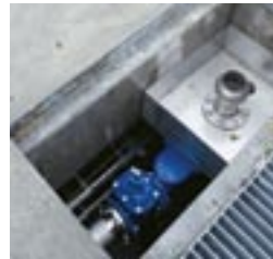
Pre-insulated Wehotek piping provides water service for ships at Vuosaari Harbour in Helsinki.
