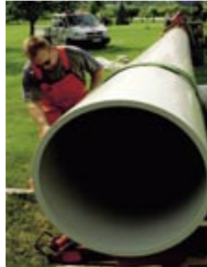
Sami Niemi preparing the relining pipe.
