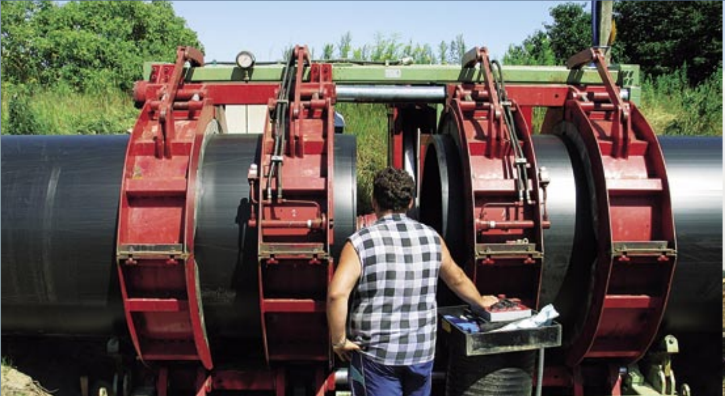
Joining the PE pipes with the KWH welding machine.
